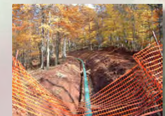
Pipeline in trench
