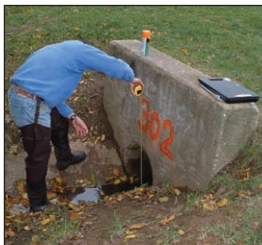
Figure 27: Measuring Outfall Diameter
