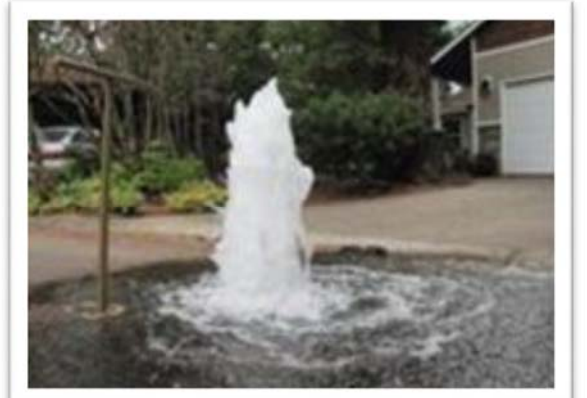
Uncontaminated Water Line Flushing
